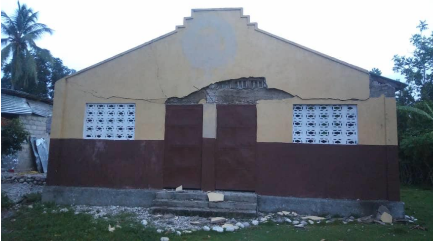
The church at Cambry was damaged by the quake.
