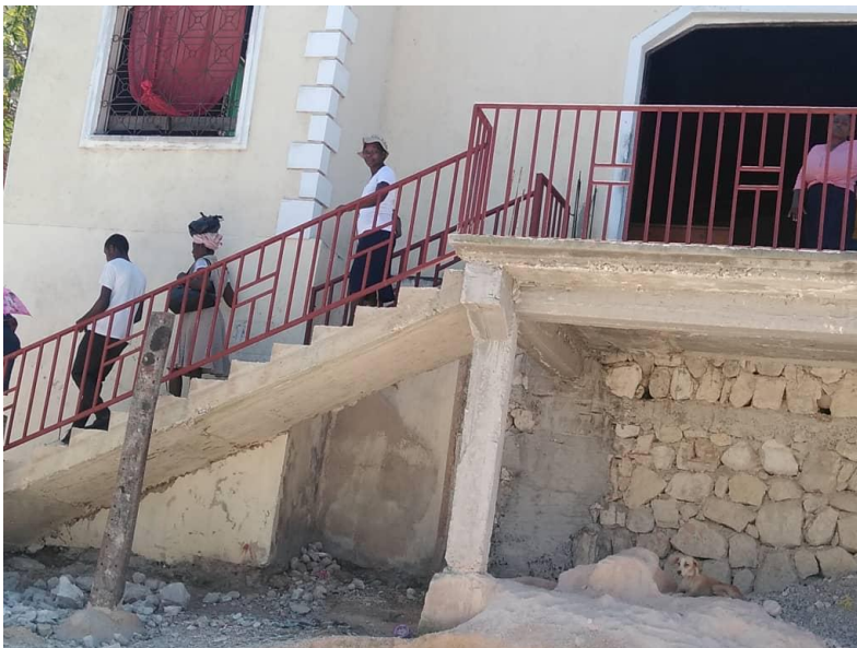
Newly reconstructed entrance to the Church at Carrefour.
