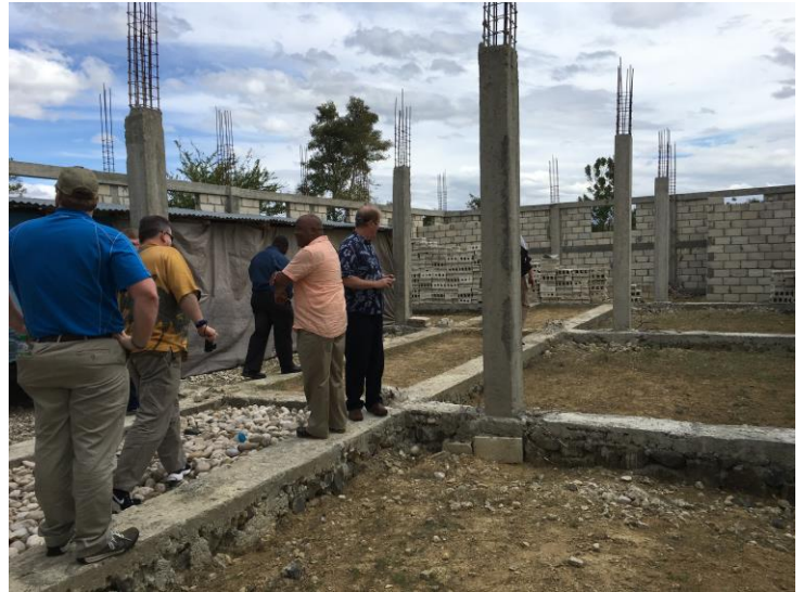
Piers and footers of the new church at Saut-d'Eau 2018
