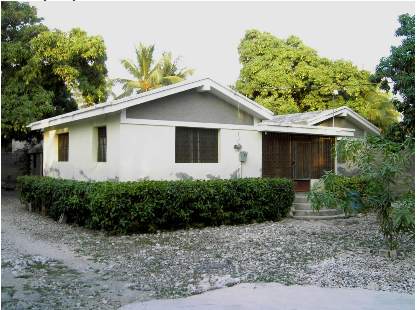
A gang of thieves broke through the concrete block wall surrounding Yvon and Claudie’s house and ransacked their home. They had people staying there and praise God, no one was injured and the thieves didn’t take anything.
